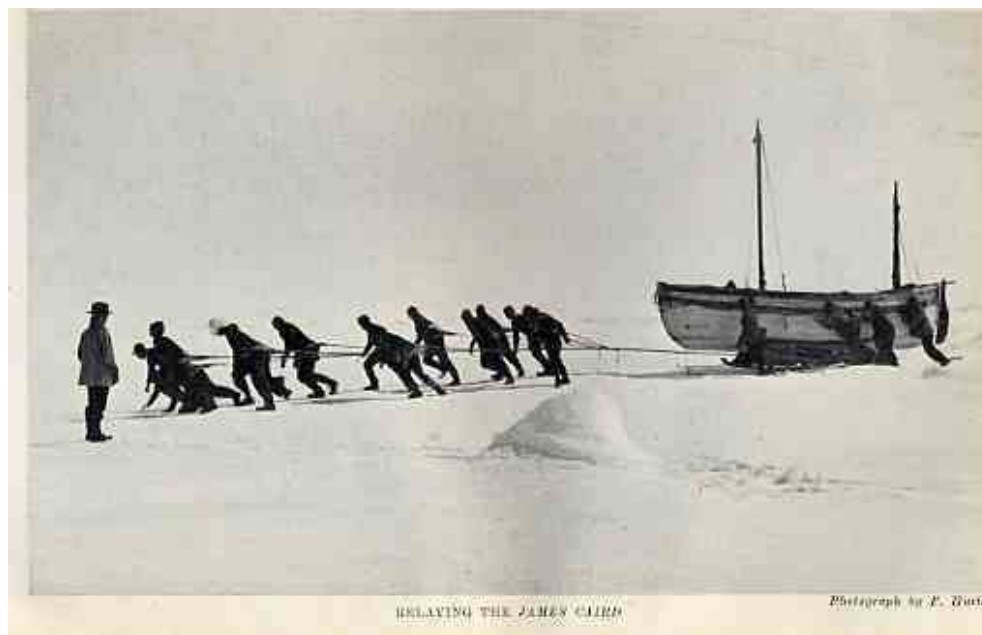
Relaying the James Caird
