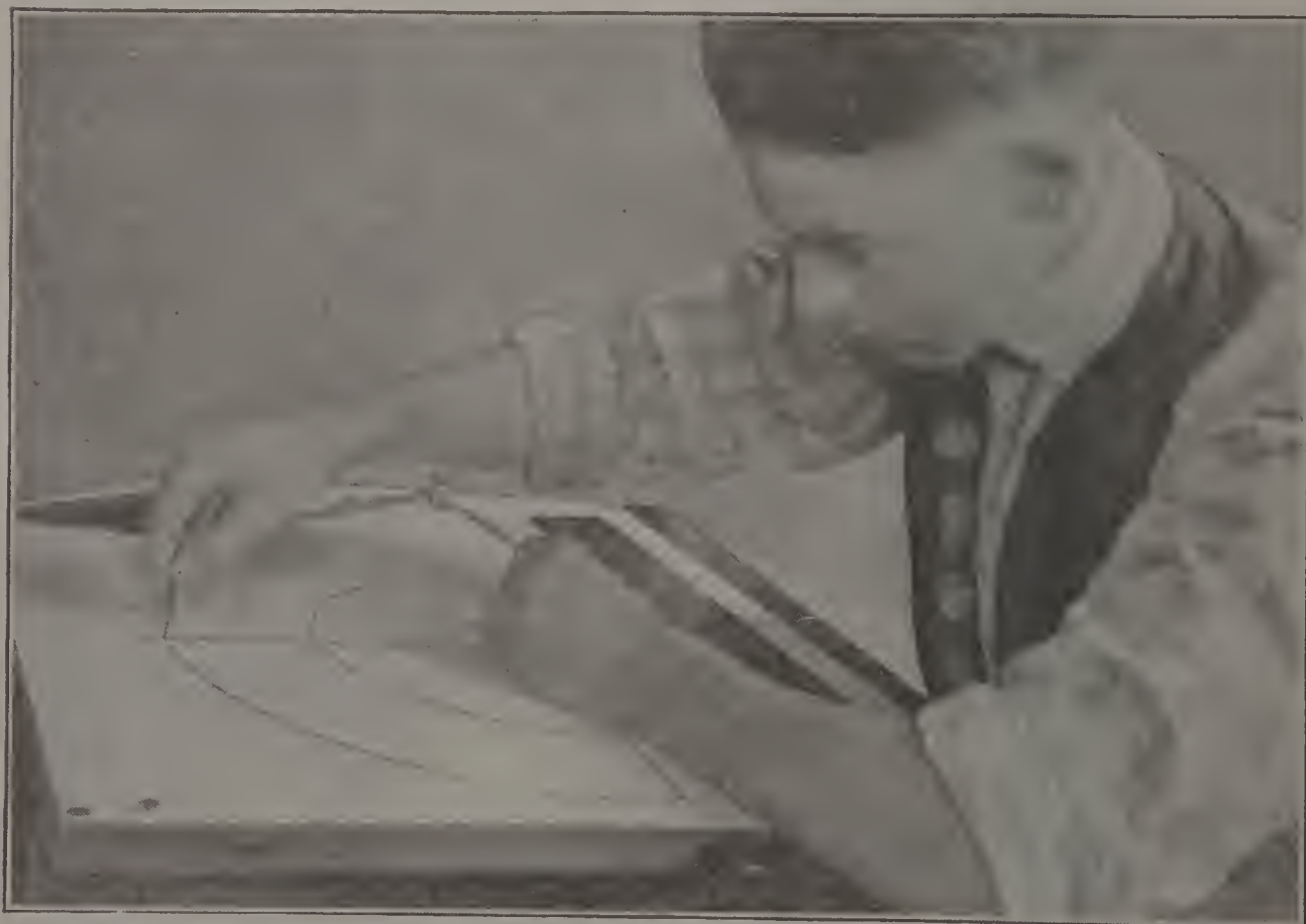
Position 6. Drawing Very Large Circle with Spread Compass and Lengthening Bar
